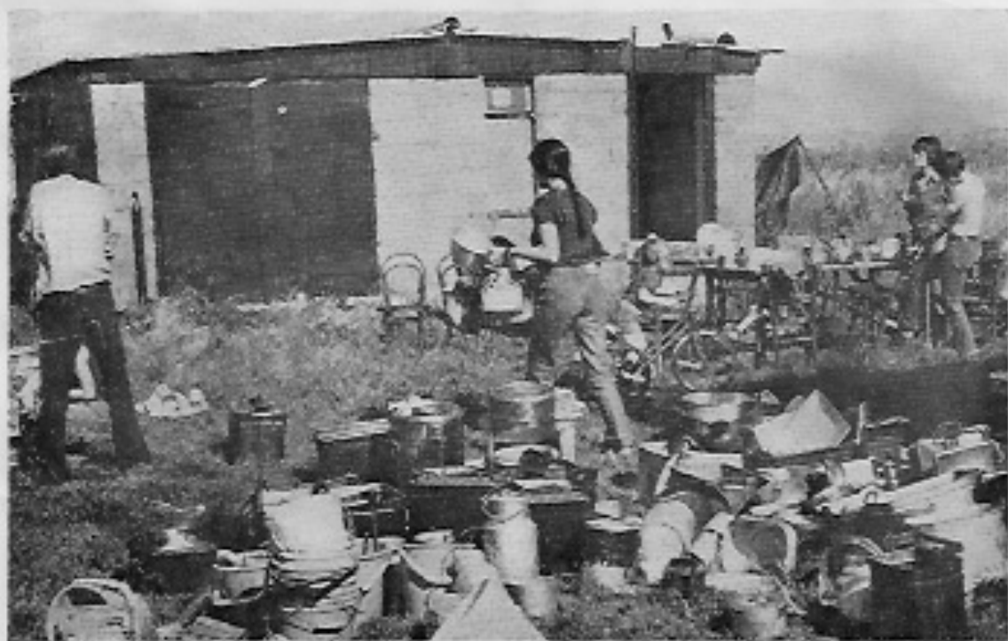
Work in progress at Haddenham
